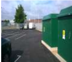
June 2017 Services upgrade
