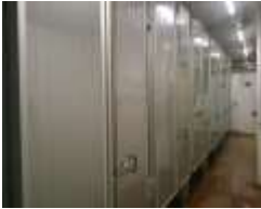
July 2017 Installation of Safechill system
