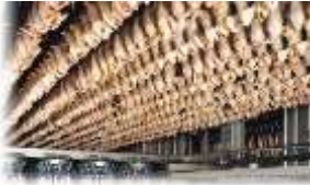
March 2018 In-line chill phase 1 installed - 15% capacity increase
