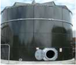
June 2018 Installation new effluent treatment plant
