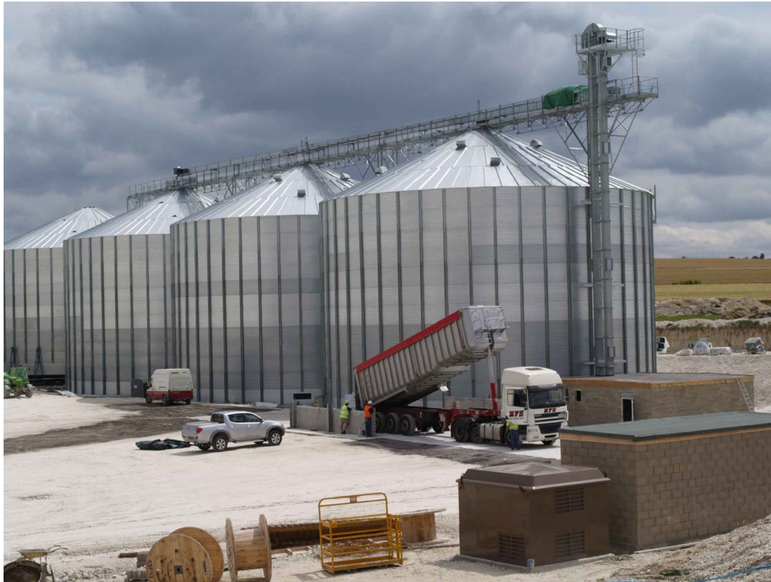
CONSTRUCTION UNDERWAY AT THE APC SITE.
